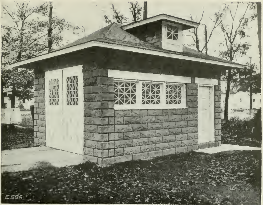
FIG. 51.—A ONE-CAR GARAGE OF CONCRETE BLOCKS.
